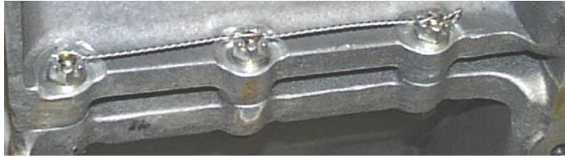
Figure 83 Safety Wire Nuts in Crankcase Oil Sump
