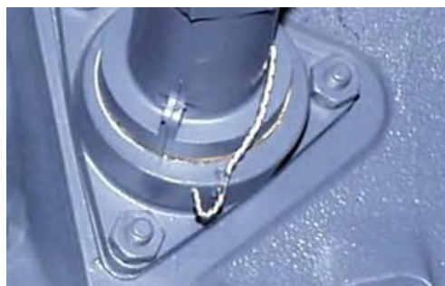
Figure 2 Safety Wire on the Oil Level Gage
