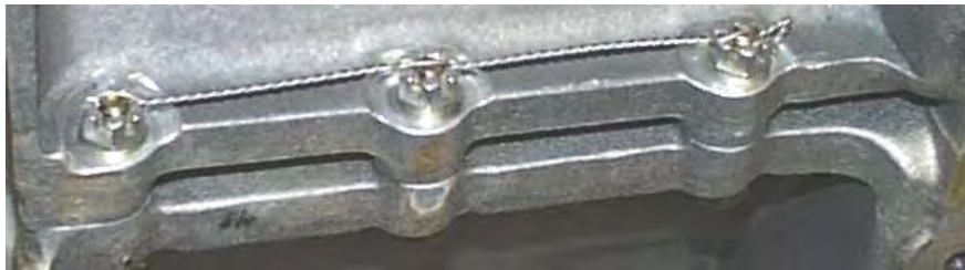
Figure 88 Safety Wire Nuts in Crankcase Oil Sump
