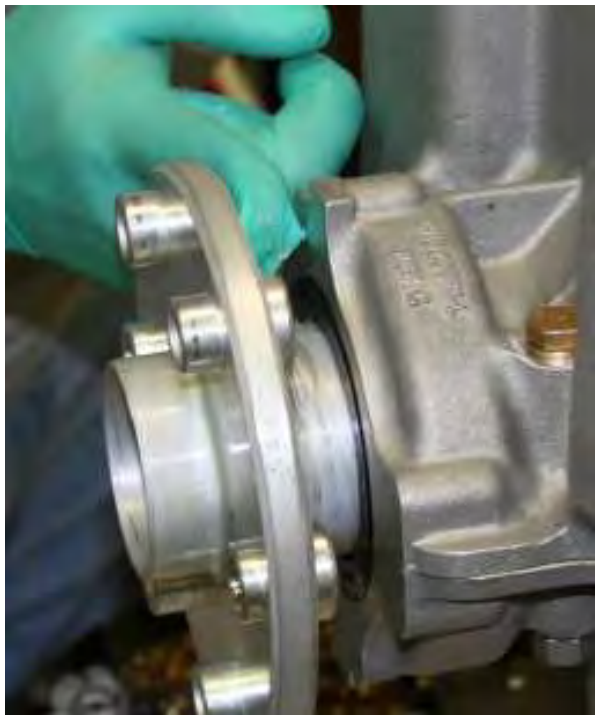
Figure 10 Spread Sealant in Gap Between Case & Seal
