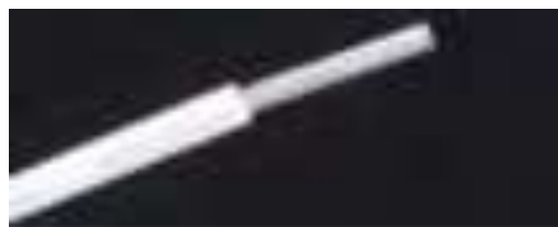
Figure 58 Properly Cut Insulation Jacket
